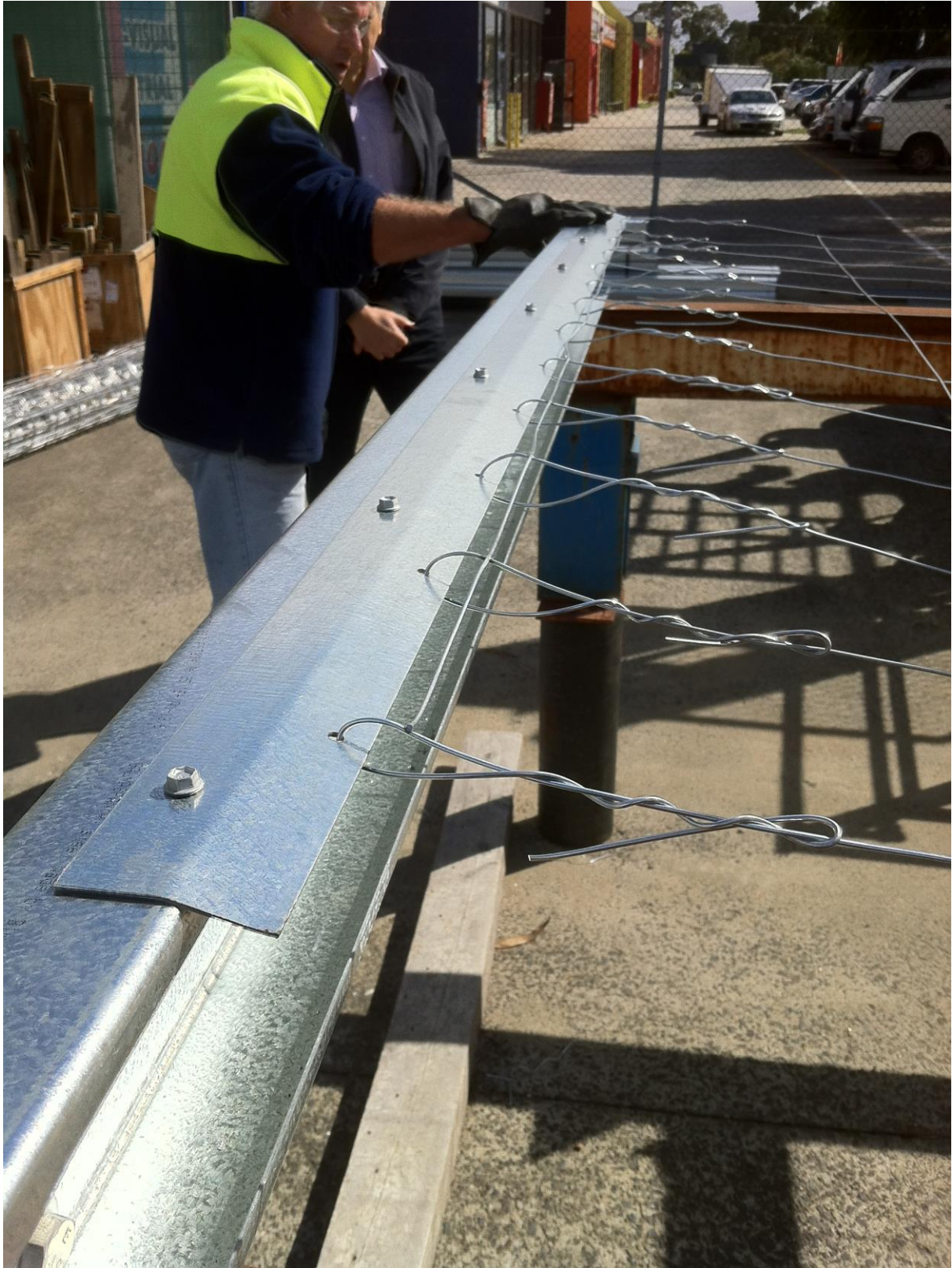
MESH STRIP INSTALLATION USING HEX HEAD TEX SCREWS (12 X 25)
